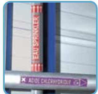
Identify pipe-lines on-site
